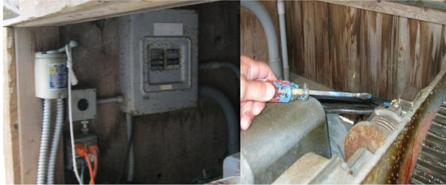
There are exposed gears that move when the winch is operated. Never allow anyone or anything to be near these gears unless the cradle is blocked and the breaker to the winch is off. Any objects or body parts pulled into the moving gears will be permanently lost.
